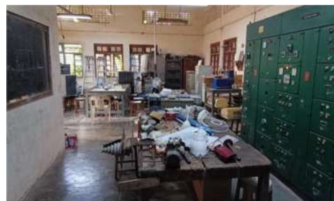
Electrical Maintenance Cell
