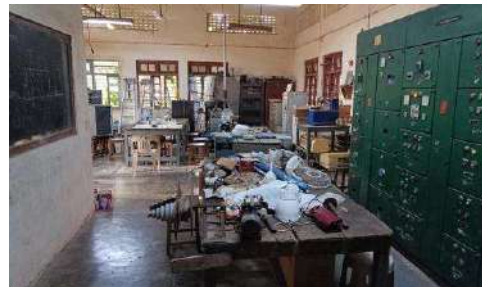
Electrical Maintenance Cell
